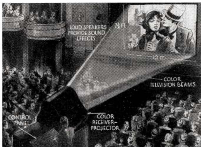
ARTIST'S DRAWING of the experimental electronic receiver-projector with which RCA demonstrated television pictures at Philadelphia's Franklin Institute last week. Screen used is theatre-type, 7½ x 10 feet. System was developed at RCA's Princeton, N. J., laboratories.
